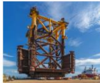
Trungnam SMC from Vietnam is a new entry this year in the T50, in at 49th place. In the pictured project it supplied Scheuerle SPMT to help Sarens load out a 4,231 tonne jacket. The load out and the load in each required 168 axle lines of SPMT and eight power pack units. Photo: Trungnam
