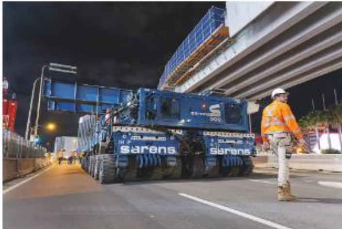
SPMTs in action during August on a Sydney project.
