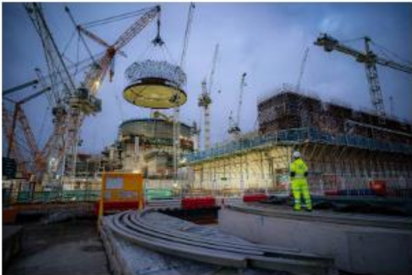
The world's largest crane, Big Carl, lifts a 340-tonne stabilizer on to Hinkley Point C's first reactor building in Somerset, as Britain looks to step up its nuclear output. AP
