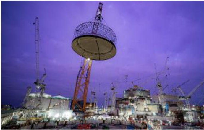
The giant crane has 10 engines and can lift up to 2,000 tonnes - equivalent to ten jumbo jets | ©2023 BBC News
