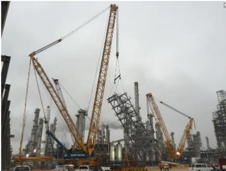
Corpus Christi polymers construction site.
