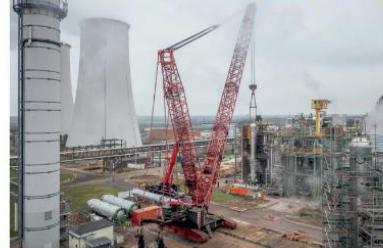
Sarens' 2,500 tonne capacity LR 12500-1.0 crawler crane at work in Germany
