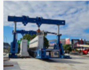
Sarens worked in the Botany Duplication using their advanced machinery
