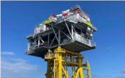
Offshore ram luffing type crane on Neart na Gaoithe (NnG) substation. (Photo: KENZFIGEE)
