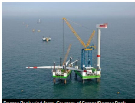
Dogger Bank wind farm. Courtesy of Sarens/Dogger Bank
