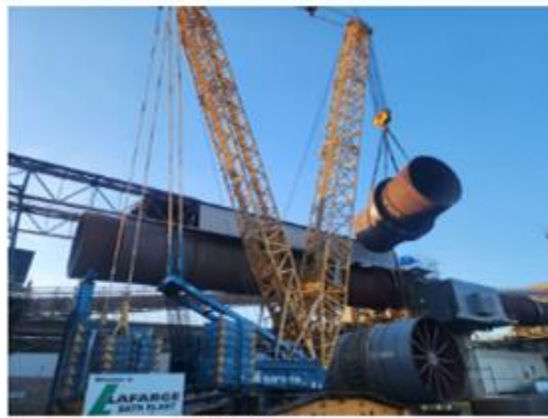
Photos courtesy of Sarens.
