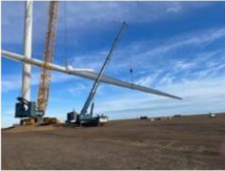
Photo courtesy of Sarens.
