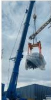
Sarens Lifting the Varian ProBeam 360.
