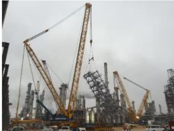
Corpus Christi polymers construction site
