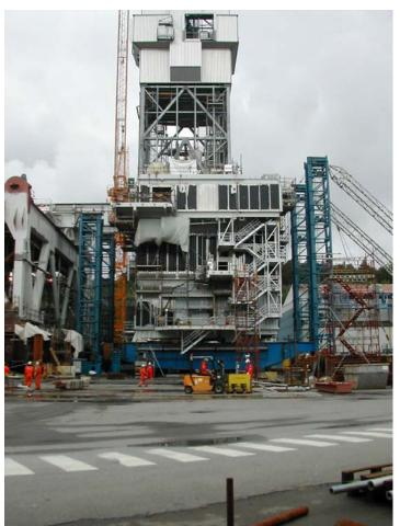
The D30 module (height 80 m - 1400 tonnes) is lifted by the SARTOWER up to a height of 22 m and skidded on top of the D40 module.
