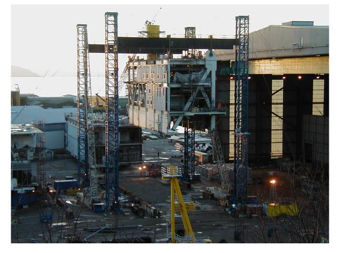
Four towers of the SARTOWER are used to lift the upper part of module D10 of the GRANE project. The lifted weight is around 1500 tonnes and the module is lifted to a height of 44 m to facilitate installation of the bottom part by means of our hydraulic trailers.
