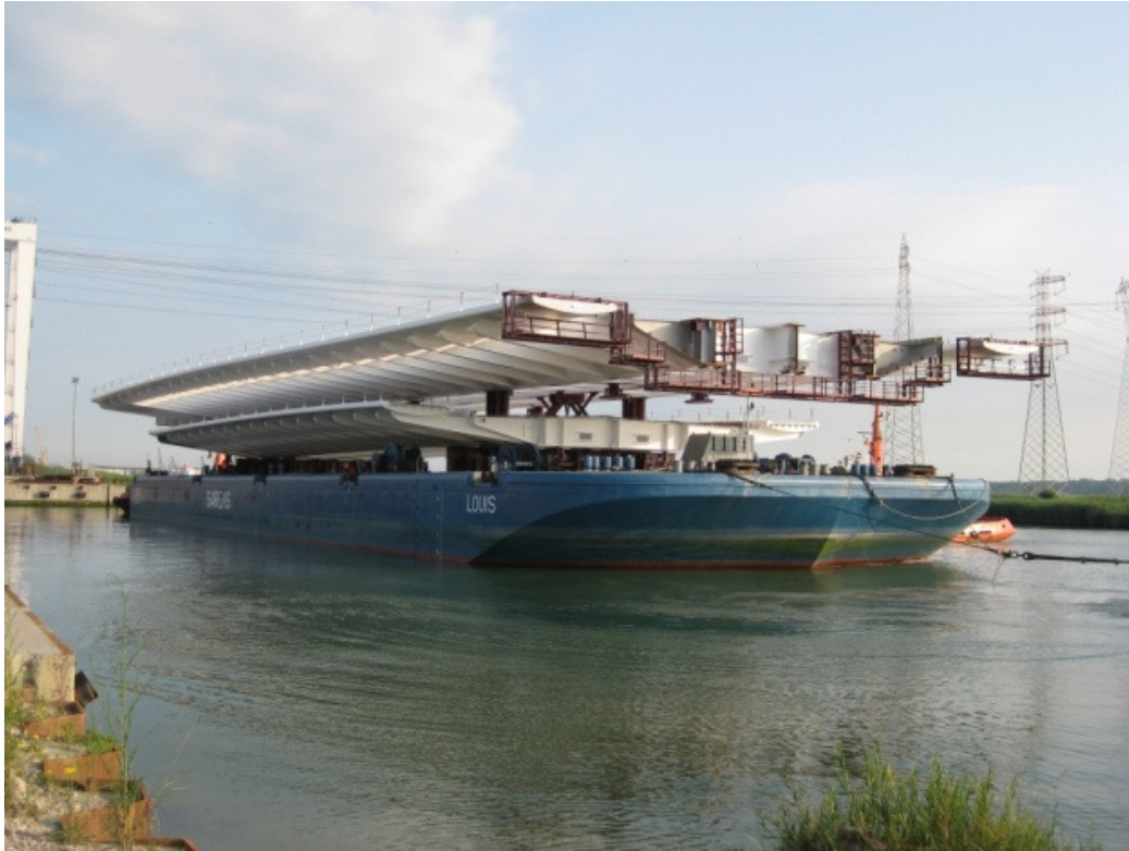
Sarens' barge Louis transports bridge parts on SPMT's
