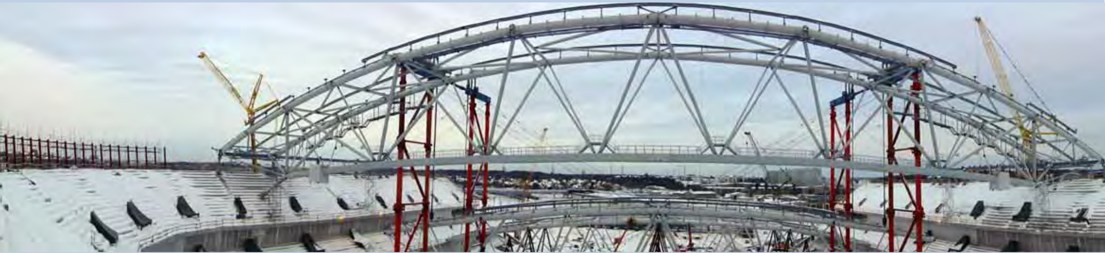
LOCATION - SOLNA - SWEDEN EQUIPMENT USED - SMLT; Strand Jacks
