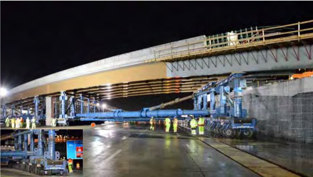
LOCATION - SALT LAKE CITY – UTAH - USA EQUIPMENT USED - 96 axle lines SPMT's and a custom-built support system
