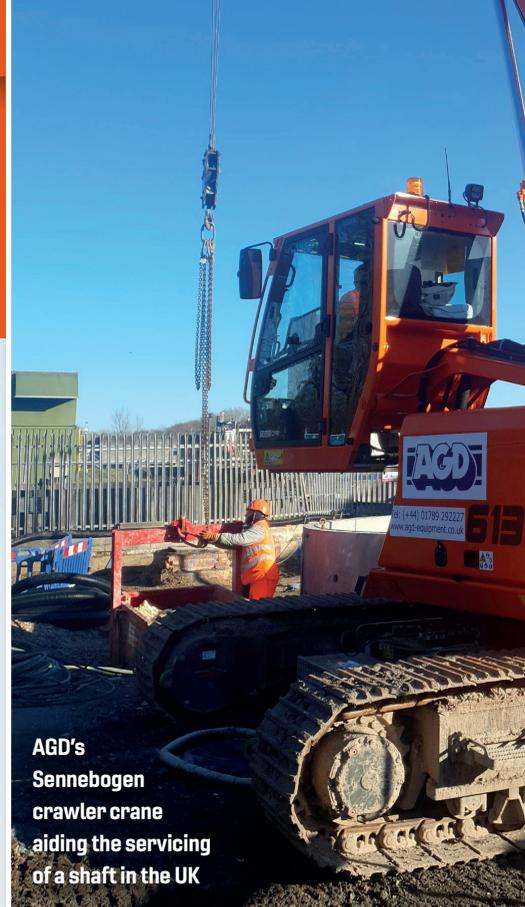
AGD’s Sennebogen crawler crane aiding the servicing of a shaft in the UK
