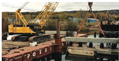
The site limitations when constructing the Highway 17 bridge over the Pays Plat River in Ontario, Canada, were overcome with Poseidon Portable Sectional Barges.
