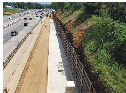
A soldier pile wall helps to minimize any damage to trees along PR-18 in Puerto Rico.
