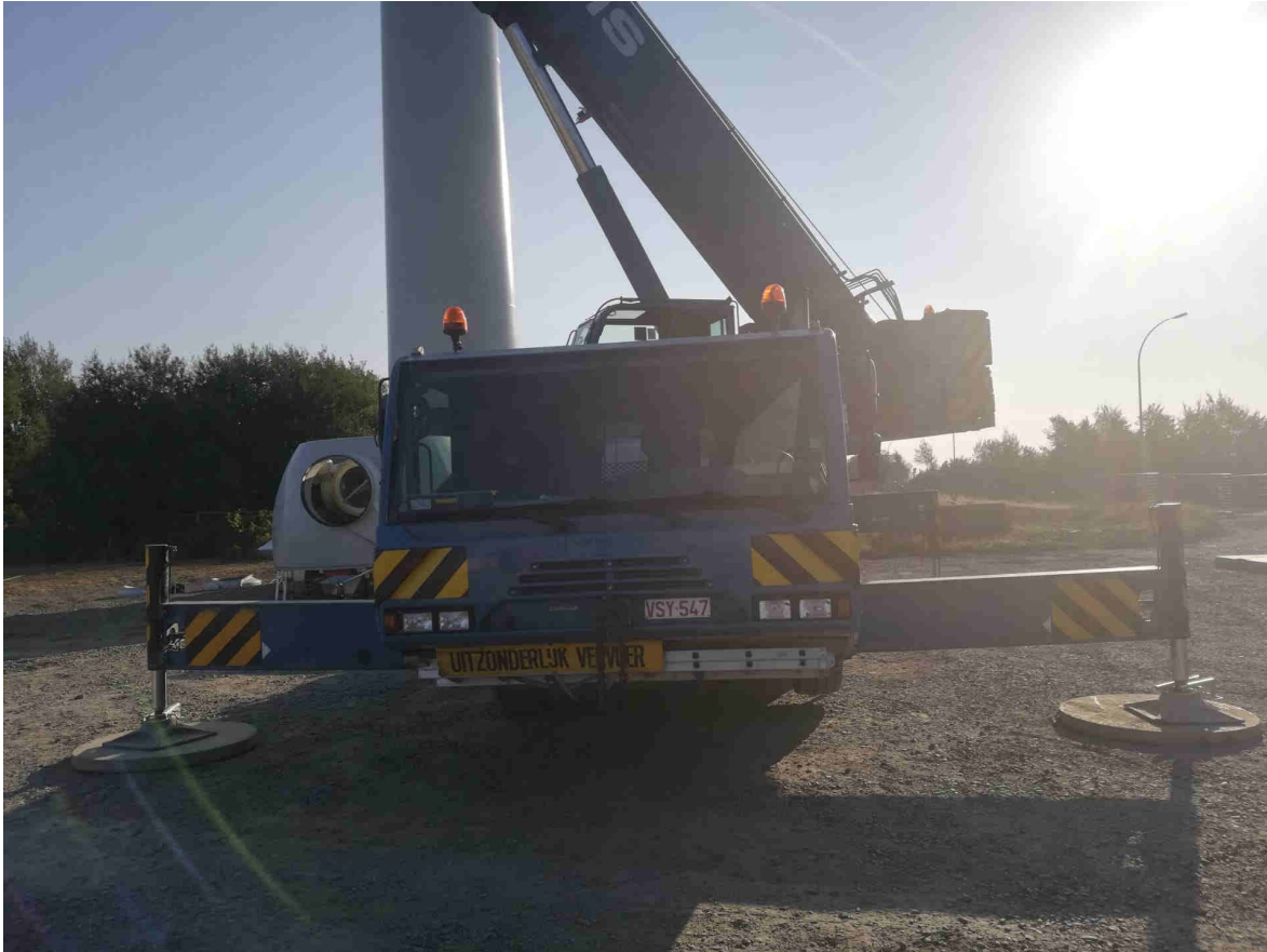
Equipment: Terex-Demag AC80-2 (2363) LOCATION: Belgium
