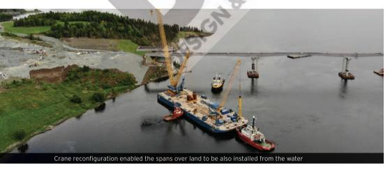
The option that was selected consisted of carrying out the whole operation over water, a method that offered the significant advantage that all the equipment required could be transported on a single barge from Sarens' headquarters in Belgium.
