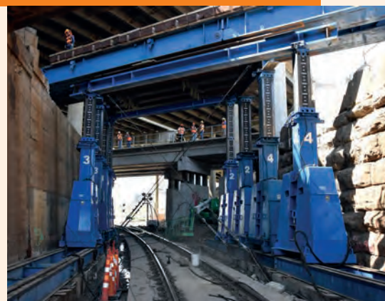
The extremely tight space meant minimal side clearances and small areas for expanding the bridges and lifting Highway 280 for its extension
