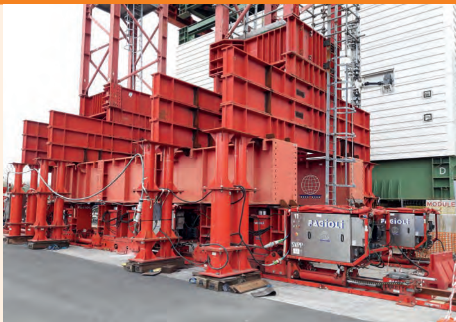
The Fagioli stacking and de-stacking operations were operationally executed in 24 hours for each single activity after a month of ground preparation and equipment assembly
