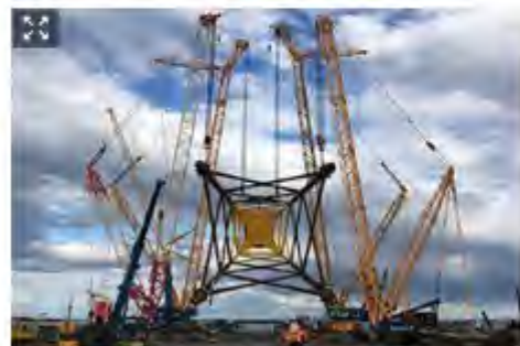
Sarens used a Demag CC 9800, CC 8800-1 and two Demag CC 2800-1s on the BiFab job
