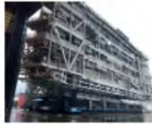
Sarens used 432 lines of Kersig K24 SPMT
