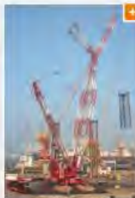
Integrated Logistics's Demag CC8500-1 lifting leg section at the Ehamia Bin Jaber Al Jalahma Shipyard complex, Qatar.
