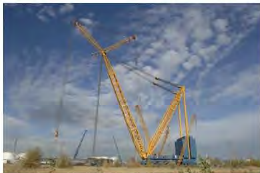
The SGC-250 lifts 5,000 tonnes.
