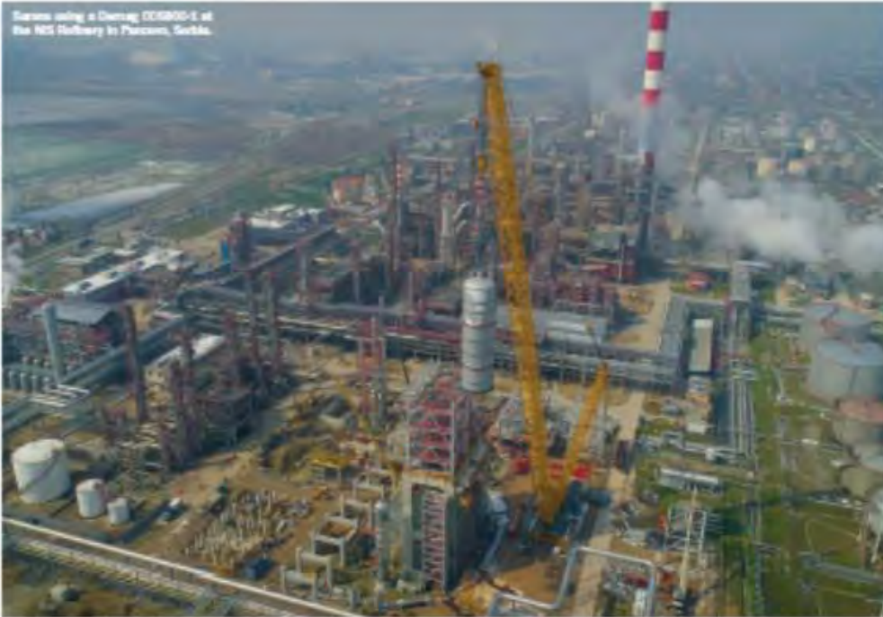
Sarens using a Demag CC8800-1 at the NIS Refinery in Pancovo, Serbia.
