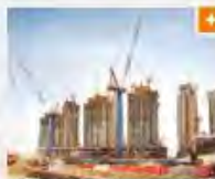
Raymond LR213 lifting crane erected at Dubai Creek Harbor.
