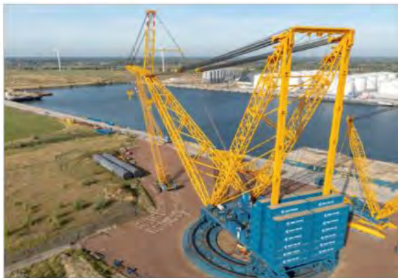
The giant crane was launched in Belgium this month and will now be transported to Hinkley
