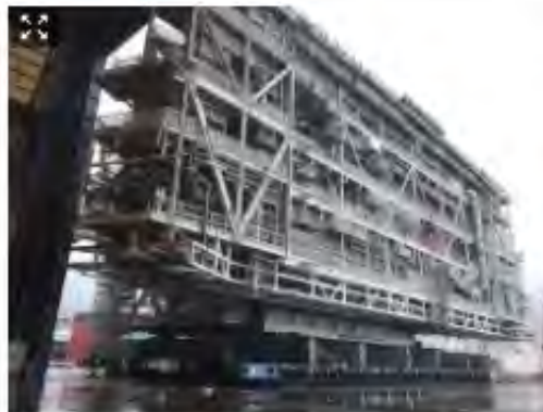
Sarens using Kamag SPMT on Johan Sverdrup oil field module
