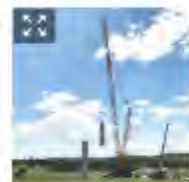
Sarens's new LG 1750 SX being used on the Sapphire wind turbine installation project in Australia
