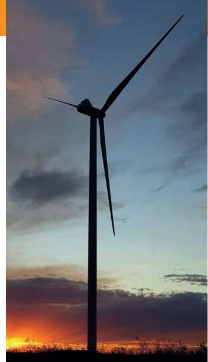
ALE provided the full-service package for the El Llano wind farm in Argentina
