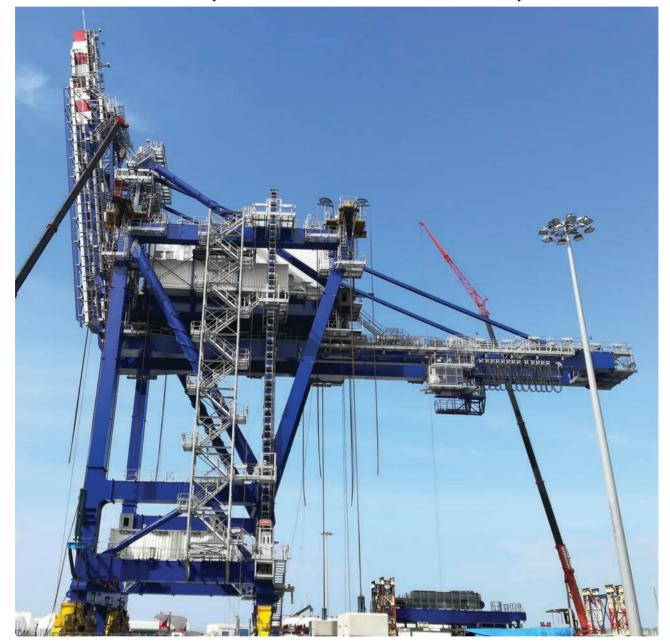
n the harbour of Bilbao, heavy lift specialist Sarens was contracted by URSSA Steel Constructions to jack-up the upper structure of a Ship Grab Unloader weighing 1100t.
