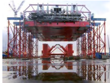
SARENS MULTI LIFTING TOWER
