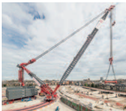
ALE has finished using its AL.SK190 crane at Earls Court in London, UK, where it says it lifted a beam weighing 1,500 tonnes – the largest single lift undertaken in UK history
