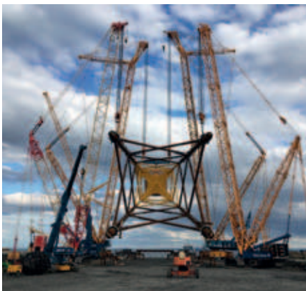
Sarens used a Demag CC 9800, CC 8800-1 and two Demag CC 2800-1s on the BiFab job
