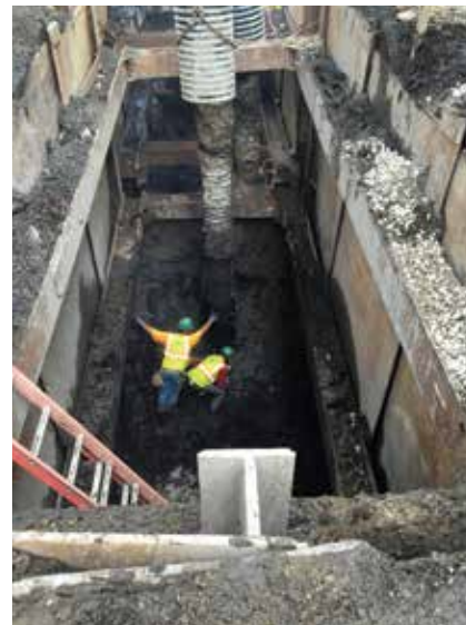
Drivecast pile provides a deep foundation solution that is cost effective and eliminates spoils and vibration during installation.
