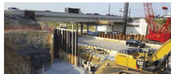
A shored MSE wall stabilized the bridge.
