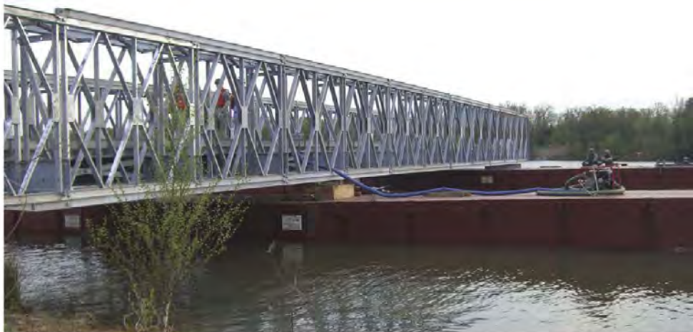
Portable sectional barges are used internationally to create temporary road bridge sections and for other applications.
