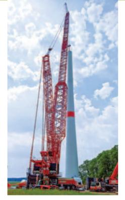
class to erect wind turbines. Liebherr says the new system can erect turbines with a hub height of up to 165 metres and component weights of up to 120 tonnes. Previously such lifts were only possible using cranes in the 1,000 tonne class or above.
