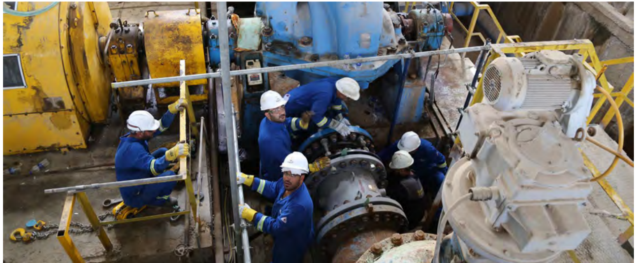
The Pipes Maintenance Team replacing the NRV – Adel Miz'el, Muhammed Fadhil, Ahmed Kareem, Ali Abed Khدير, Layth Kareem, Mohammed Tahssen, Mohammed Baker
