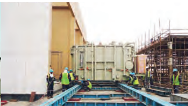
In-House Developed Jacking & Sliding Techniques
