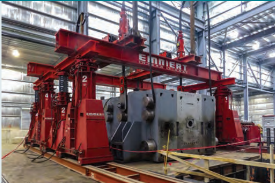
To lift and set the final press crown, only 6 inches (150 mm) of clearance was available from the top of the strand jack guide to the bottom of the roof structure
