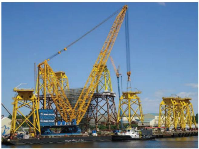
**SARENS** team offloading jacket top pieces (397 ton each) from the **ROROPONTON 4** using their **SGC-120** (**Big Benny**) **crane**. The load was smoothly maneuvered around the **MULTRATUG 3** at the **Smulders jacket yard** in Wallsend (UK). The SARENS crane is fit with a 130 meter main boom and has **3600 ton counterweight**. The hock block weighs 79.4t (!) **and setting down this jacket part 120 meter away is not even a problem - <b>Photo : John Smith** ©
