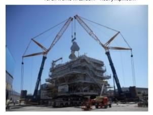
In order to avoid a potential overload on one of the cranes, Sarens positioned a 160-tonne capacity swivel beam in between the spreader bar and the cranes' hook blocks.
