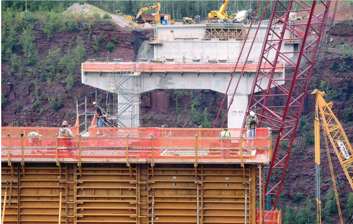
Workers on top of the the east pier of the U.S. Highway 53 bridge being built across the Rouchleau pit work on a temporary platform. The pier stands 185 feet above the pit's water. Steve Kuchera / skuchera@duluthnews.com
