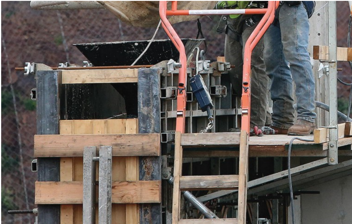
Workers prepare to pour concrete for the west abutment of the U.S. Highway 53 bridge being built across the Rouchleau pit. Steve Kuchera / skuchera@duluthnews.com
