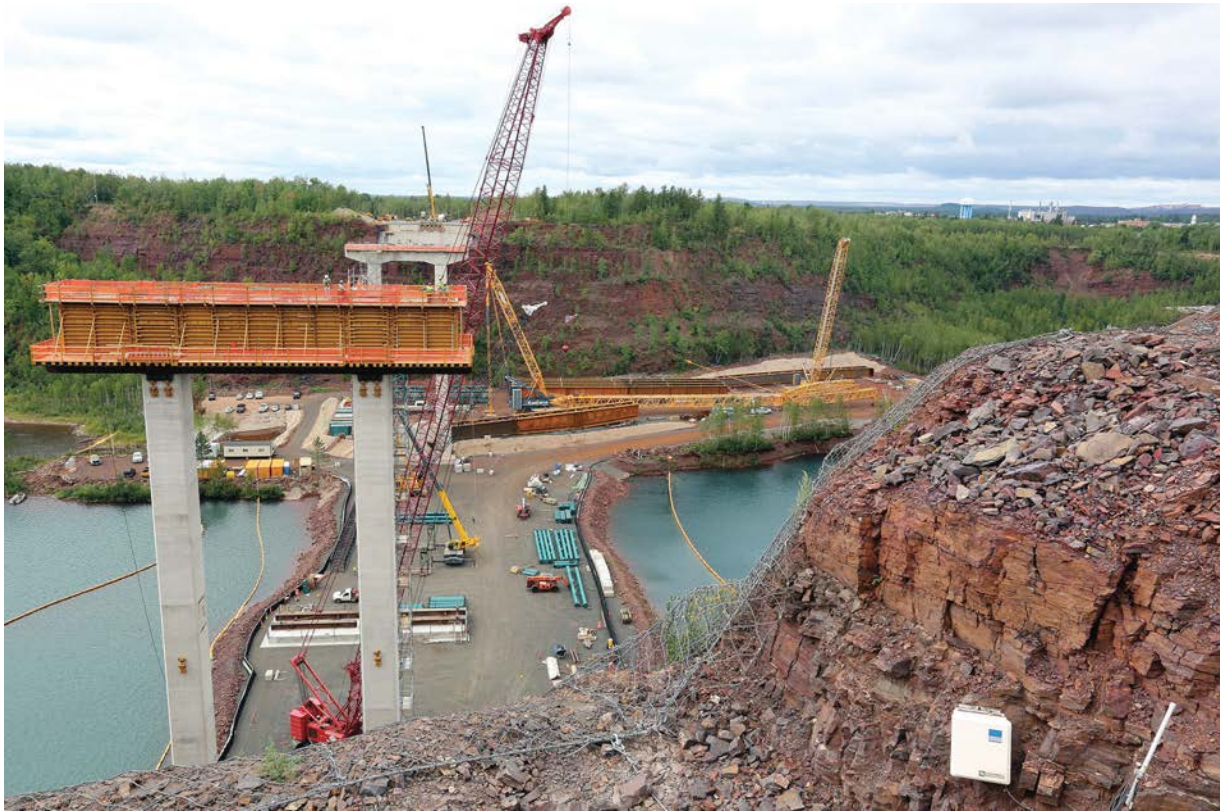
Work is moving along on the U.S. Highway 53 Bridge over the Rouchleau pit in Virginia. Both piers are finished, with the east pier (foreground) raising 185 feet above the water. Workers will begin raising the bridge's beams next month. Steve Kuchera / skuchera@duluthnews.com
