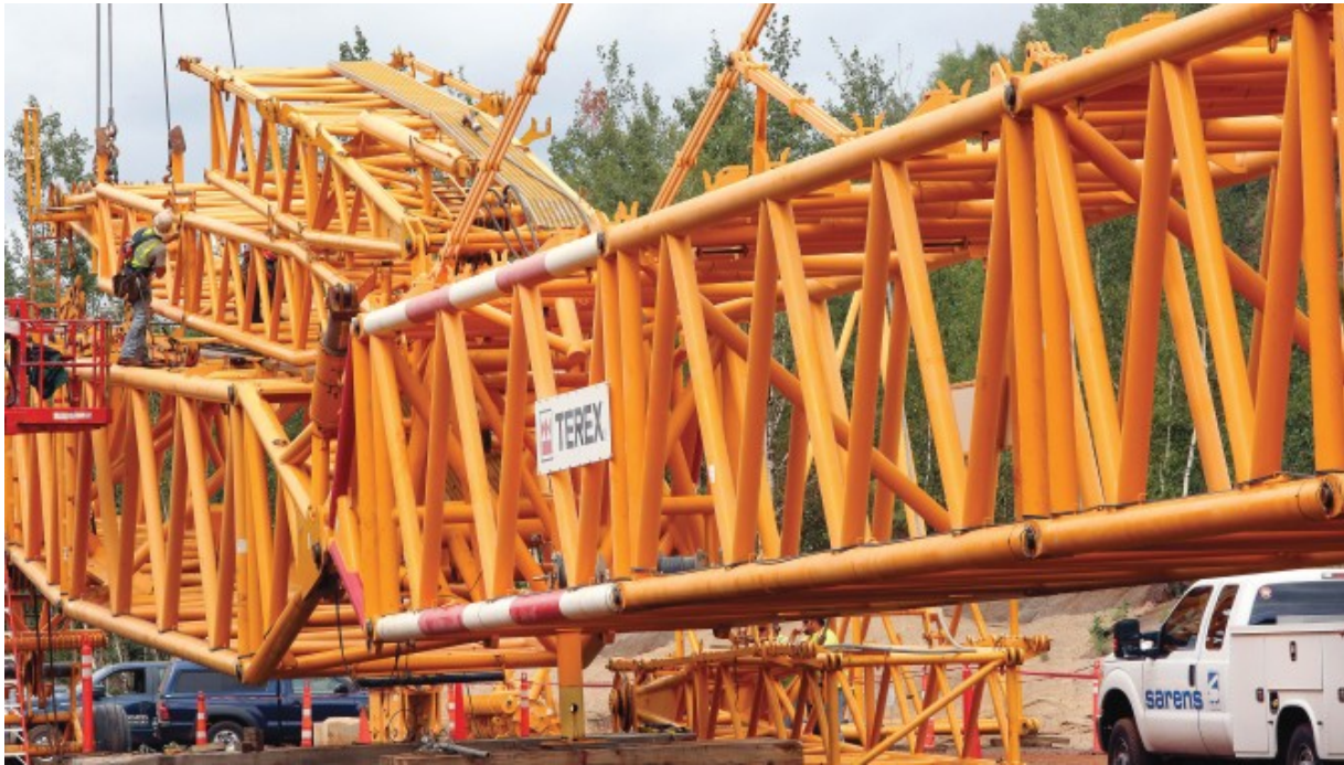
Workers and a truck are dwarfed by the boom of the crane that will lift beams into place on the U.S. Highway 53 bridge being built across the Rouchleau pit. Steve Kuchera / skuchera@duluthnews.com
