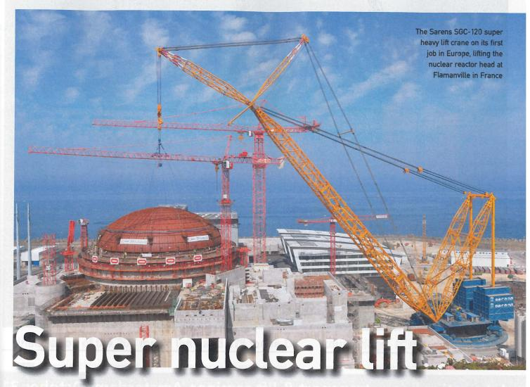
International lifting and transport specialist Sarens from Belgium used its 3,200 tonne capacity SGC-120 super heavy lift crane for a lift weighing hundreds of tonnes - at well over 100 metres radius - on a nuclear power plant project in France. IC reports
