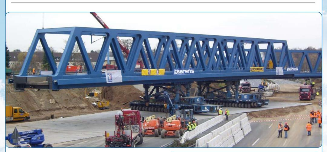
As a measure to the increasing traffic around the city of Köln, additional lanes were added to the motorway, causing several bridges to be replaced. During 2 consecutive weekends, both 750 ton spans were successfully moved in place.
