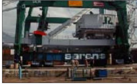
For this project in Rouen, Sarens SPMT's and ballasting equipment were used to unload two container cranes, with a total weight of 850 tonnes, from a sea-going barge. After careful preparation, the cranes were then self-erected using a combination of twelve strand jacks. By positioning the strand jacks on top of the crane legs, the superstructure — which
