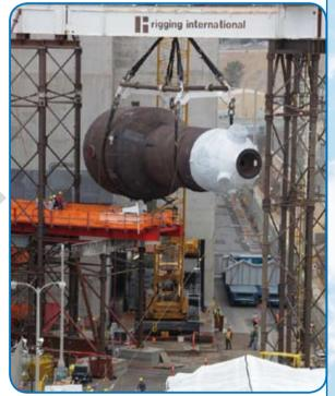
plant site. For the placement of the two new steam generators, the same equipment was utilized in reverse fashion to complete the final installation.
