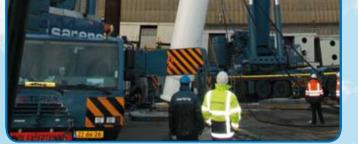
For the second time Sarens installed 8 boiler-units (weight: 125 to 175t) in the "Vasilikos" power plant. The boiler-unit first had to be lifted using a 300t crane and a combination of "Stretch - SPMT - Gantry - 2 Strand Jacks 100t" on top of the skidding beams that were installed on a 6m higher level. From this position the boiler-unit was lifted 28m from horizontal to vertical position using 2 Strand Jacks 100t and a special tailframe placed on the Sarskidsystem.
