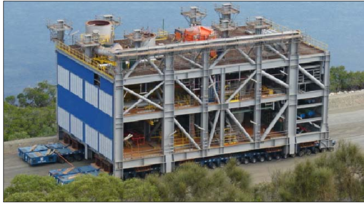
Client: Hatch - Technip Location: Koniambo - New Caledonia Weight: 3900 T
