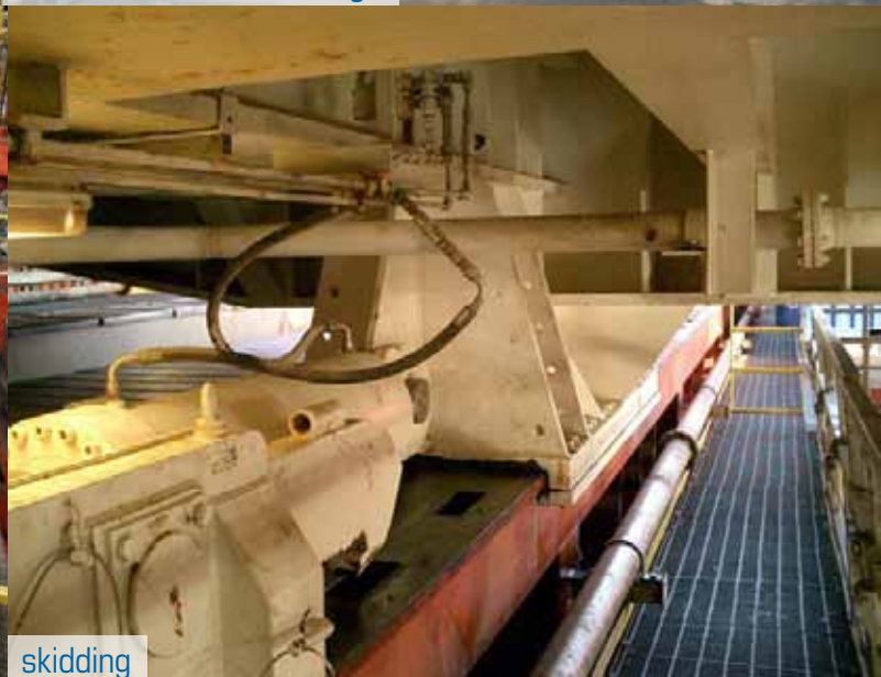
module lift skid onto barge
