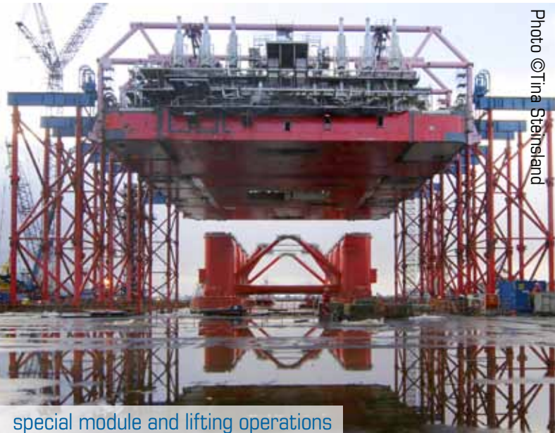
module lift skid onto barge
