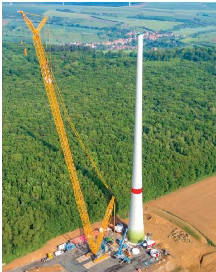
between turbines. Once the crane is set up on the outriggers at the next turbine, the trailer can then go back to move the fully-rigged Superlift mast system in one go.
