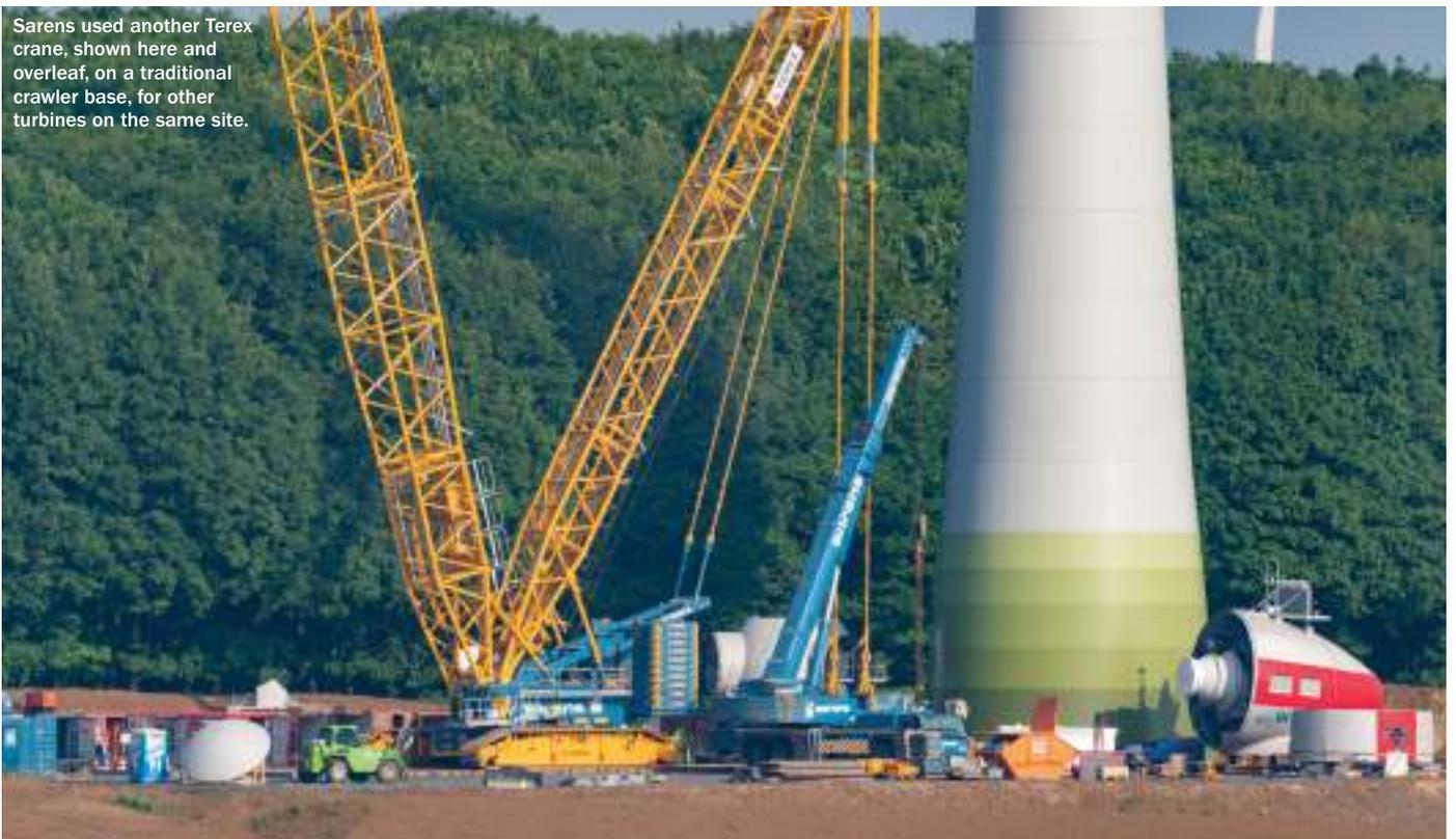
*Sarens has demonstrated the advantages of its new 'mobile' pedestal crane, the Terex PC 3800-1, on a wind farm project in Germany. The crane was used to erect three 159m wind turbine towers.*
