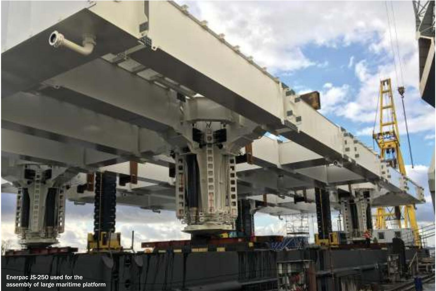
Enerpac JS-250 used for the assembly of large maritime platform
