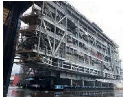
Sarens used 432 lines of Kamag K24 SPMT
