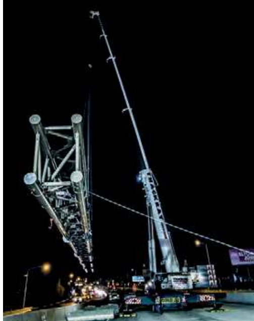
Thackray Crane Rental was called to help install a new highway signage truss over Interstate 95 in Philadelphia, USA. The lift required a 400 tonne capacity Liebherr LTM 1400.7.1
