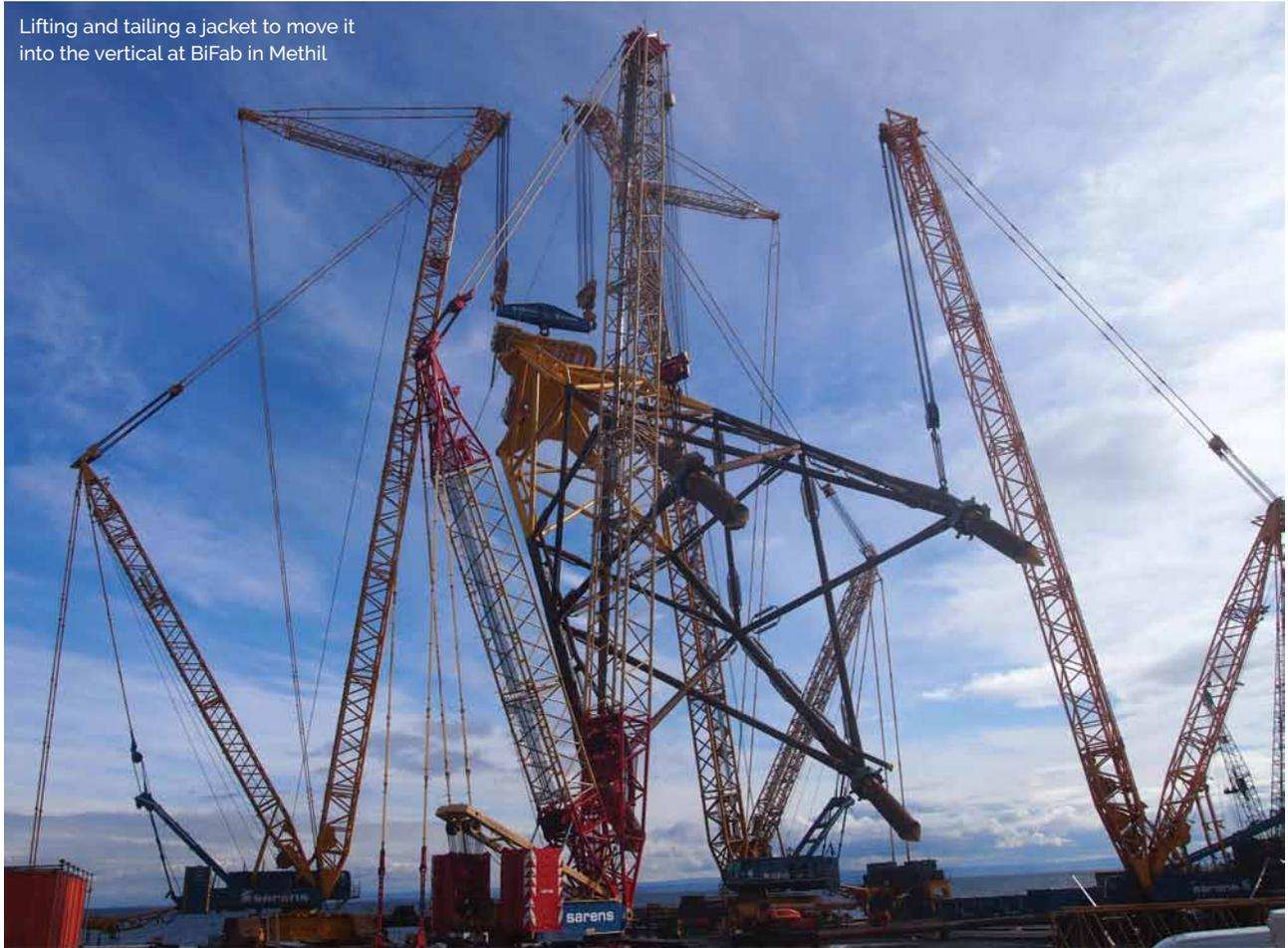
The current stage of the project will see the 86 jackets, each weighing around 1,000t, installed on top of the foundation clusters. At sea, these will be installed by the heaviest offshore crane in Seaway's fleet, the Oleg Strashnov.
