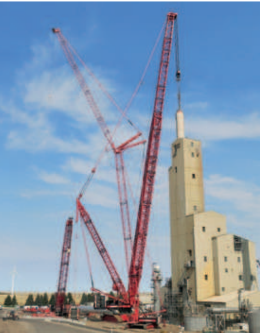
Mammoet used its Liebherr LR 11350 for an R-101 vessel replacement job in Southern Alberta, Canada
