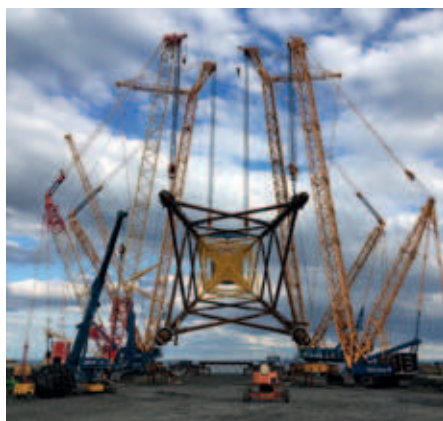
Sarens used a Demag CC 9800, CC 8800-1 and two Demag CC 2800-1s on the BiFab job
