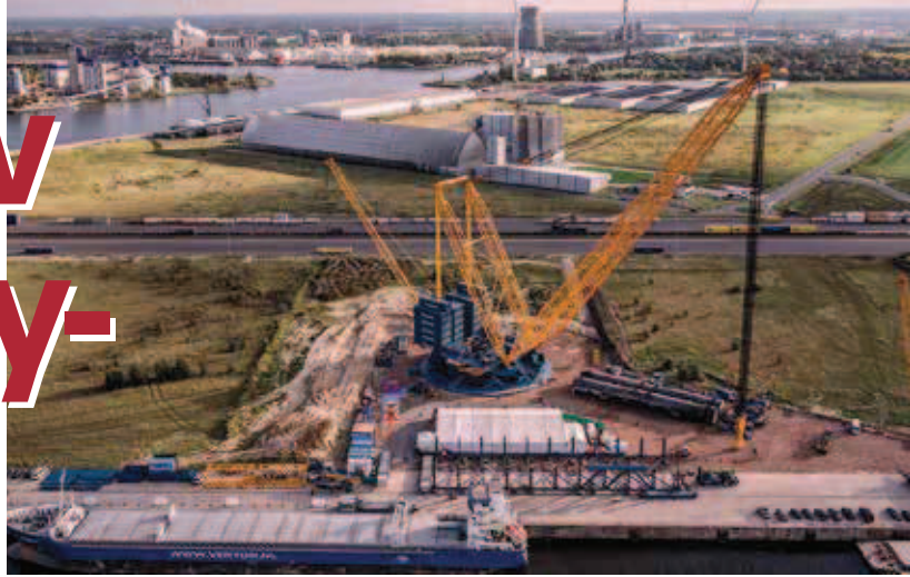
40 counterweight containers each weigh 100 tonnes
