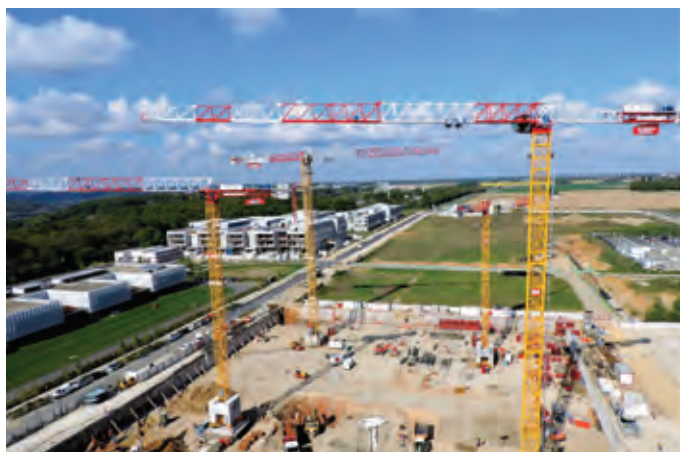
Six Raimondi flat top towers installed by GP Mat International in Saclay, Paris, France
