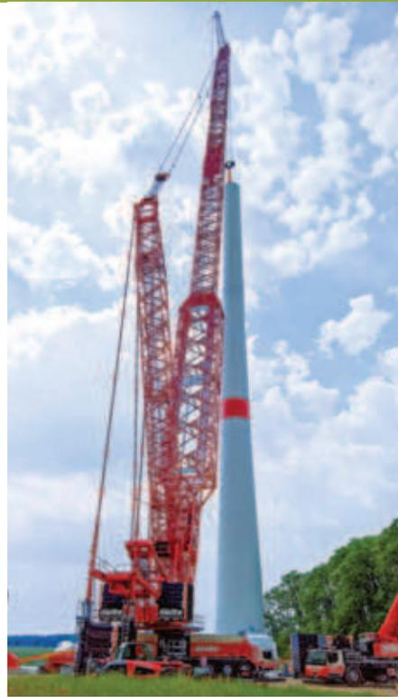
class to erect wind turbines. Liebherr says the new system can erect turbines with a hub height of up to 165 metres and component weights of up to 120 tonnes. Previously such lifts were only possible using cranes in the 1,000 tonne class or above.
