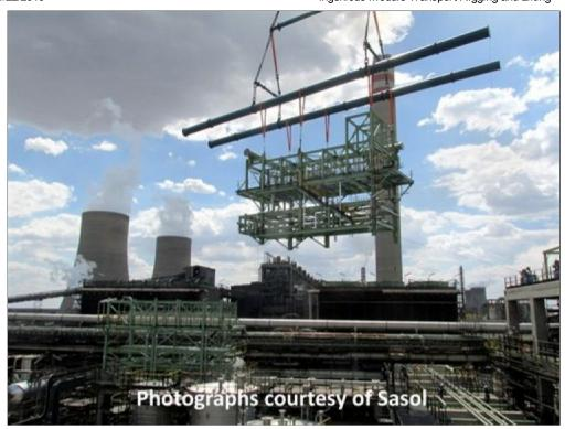
Sarens in South Africa was awarded the contract for the transportation and rigging of 24 modules encompassing an estimated design mass in excess of 1,500 Tons, the largest being 248 Tons. This was undertaken in alignment with Sasol's Integrated Management Team's (Sasol-IMT) requirements.
