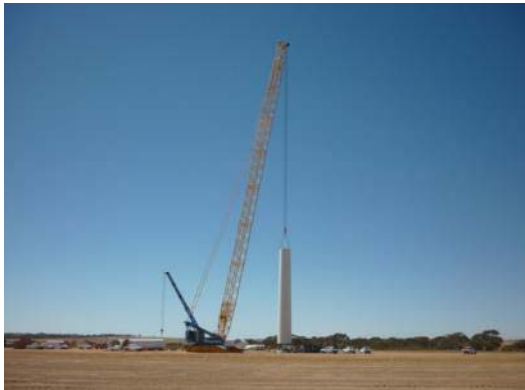
Preassy crane LR1350LN
