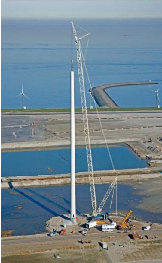
Vestas Benelux Eemshaven V90 (3MW) / 100m
