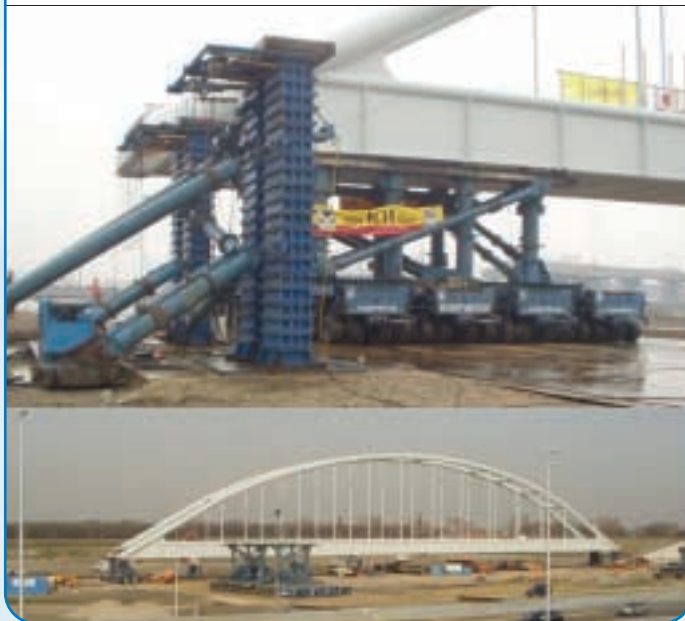
New railway bridge over highway A12 in Nootdorp (NL)
