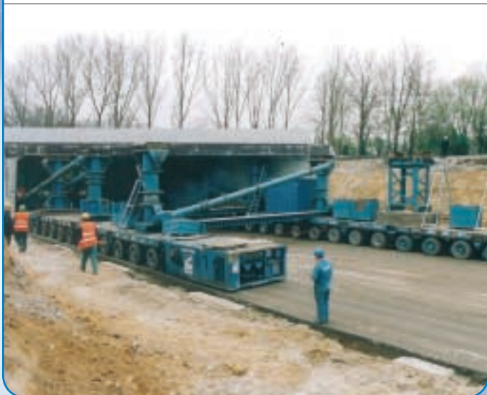
Positioning of 2 concrete bridge sections in Wommelgem (B)
