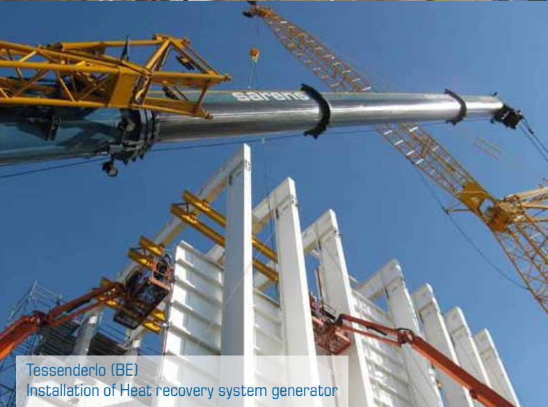
Tessenderlo (BE) Installation of a stack
