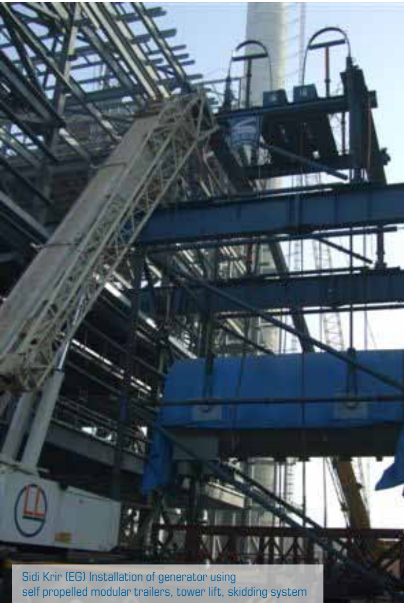
Cairo West (EG) Installation of generator using self propelled modular trailers, skidding system, strand jacks
