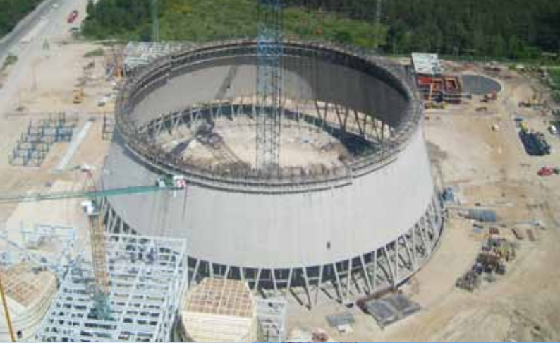
Belchatow (POL) : Cooling tower construction Heavy Lift tower crane Free standing up to 100m
